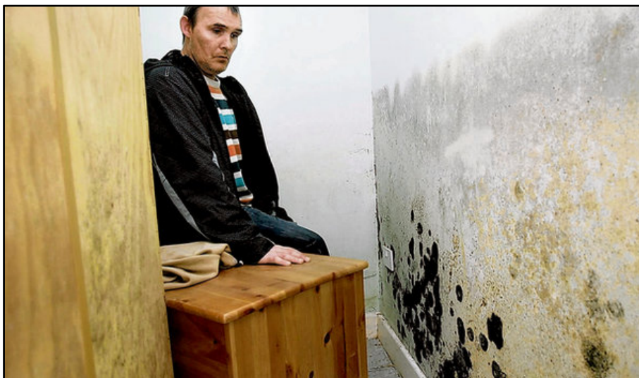
Figure 5 Mould visible on the walls in Balgaddy (Holland, 2011)
